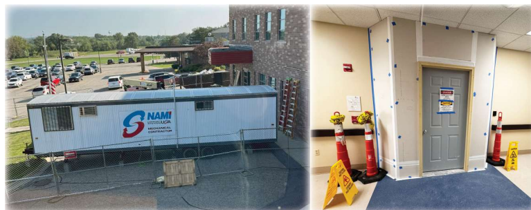
Mile Bluff's "old" Emergency Department is officially under construction! Crews are in the thick of demolition.
